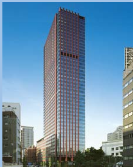
Sumitomo Fudosan Mita Twin Building West
