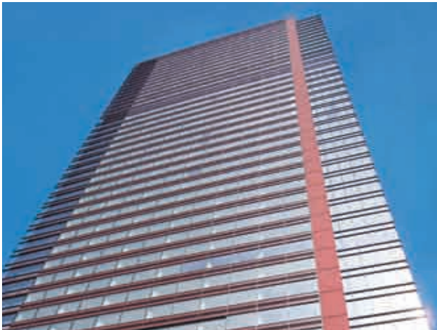
Sumitomo Fudosan Mita Twin Building West
