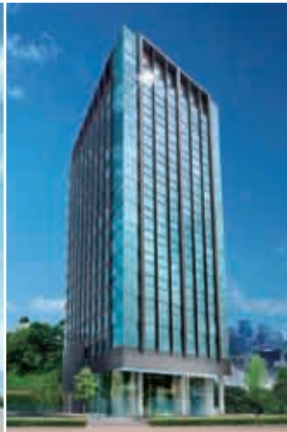
Chiyoda First Building South
