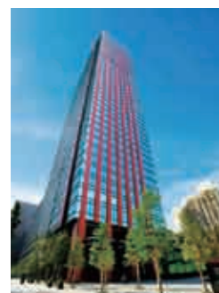
Sumitomo Fudosan Mita Twin Building West
