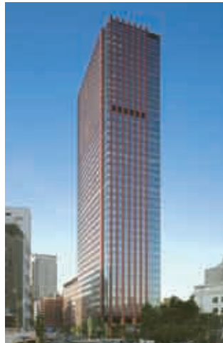
Sumitomo Fudosan Mita Twin Building West
