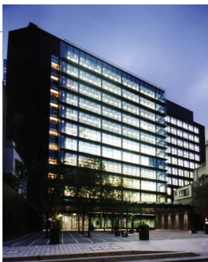
Sumitomo Fudosan Shin-Akasaka Building
