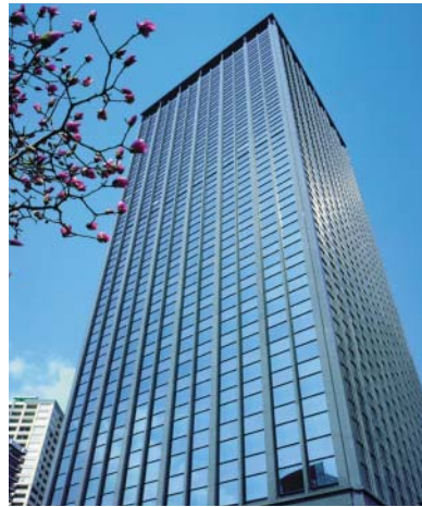
Chiyoda First Building West
