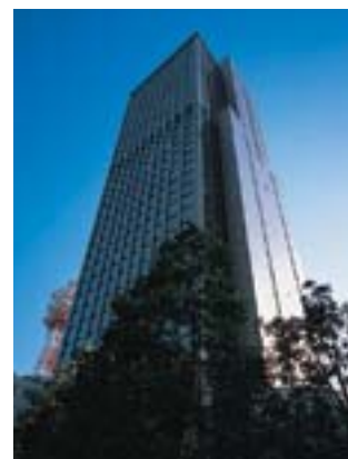
Shibakoen First Building
