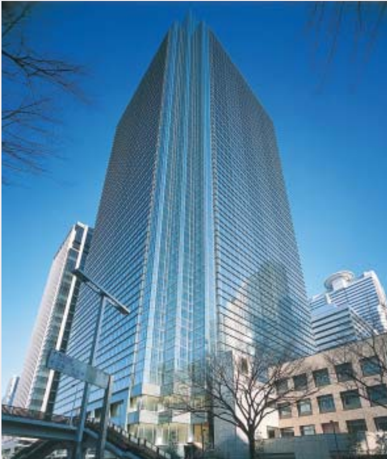
The Sumitomo Fudosan Shinjuku Oak Tower (Nishi-Shinjuku 6-Chome Redevelopment Project) [Completed Jan. 2003]
