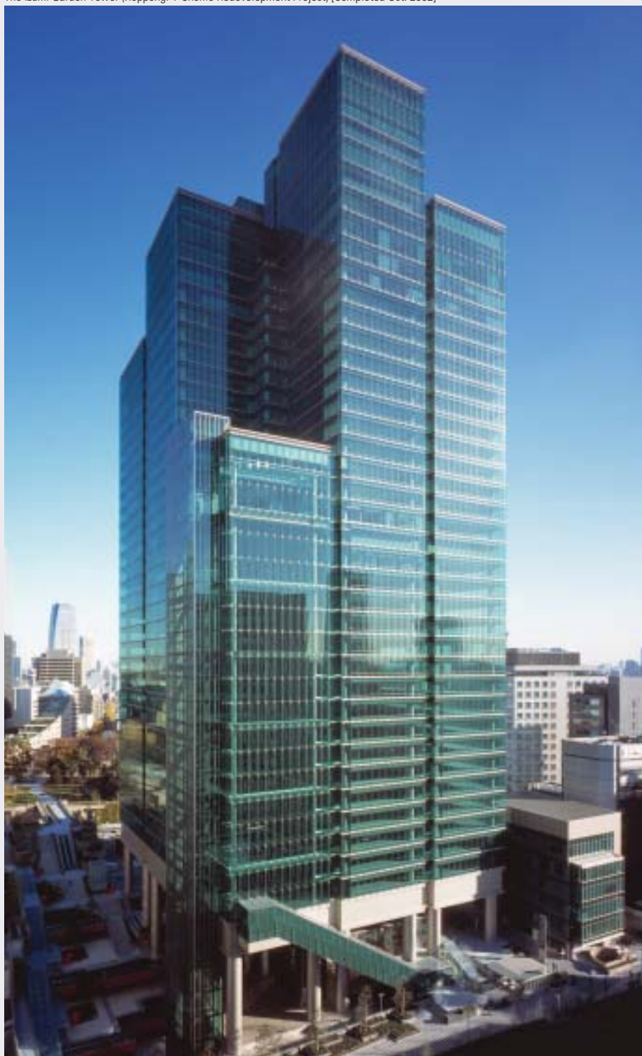
The Izumi Garden Tower (Roppongi 1-Chome Redevelopment Project) [Completed Oct. 2002]
