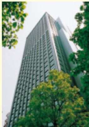
The 100-meter high La Tour Shibakoen condominium offering secure and luxurious residences.
