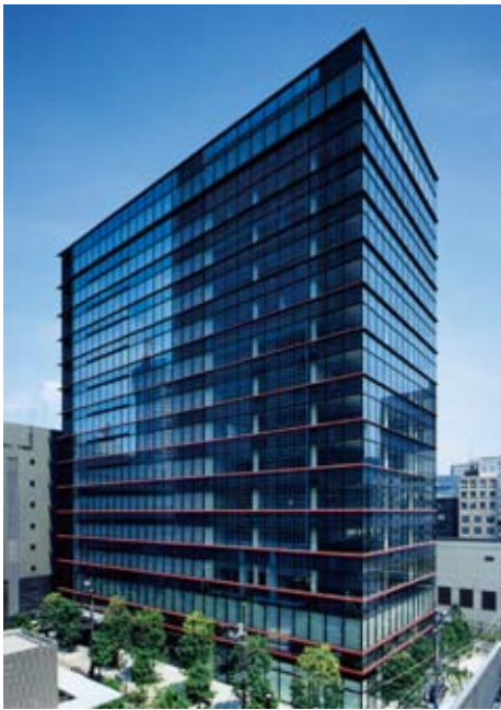
Sumitomo Fudosan Iidabashi Ekimae Building (Completed May 2008)
