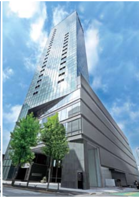
Sumitomo Fudosan Nishi Shinjuku Building No. 5 (Completed May 2008)
